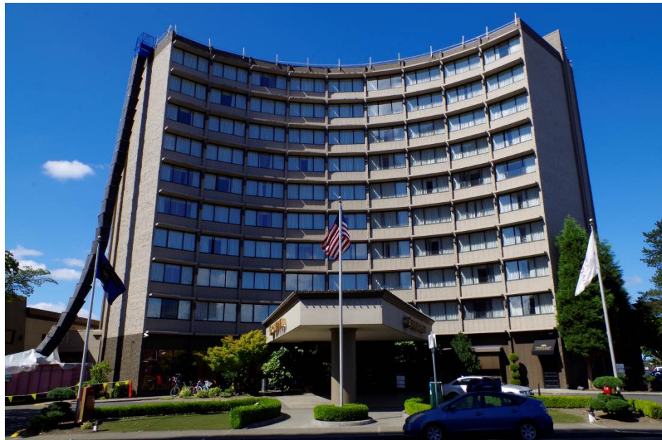
Photograph 2. The TraveLodge at the Coliseum west elevation, looking southeast
